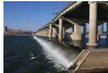
Small-scale hydro power station
