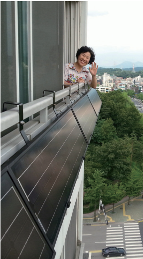
Mini PV System for Apartment
