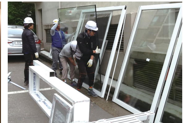
Window Reinstallation for BRP
