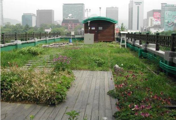
<Figure 4> Green Garden of Seoul City Hall Annex
