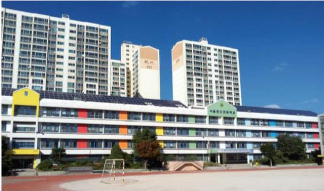
Figure 10. Solar Panels Installed on a School Roof
