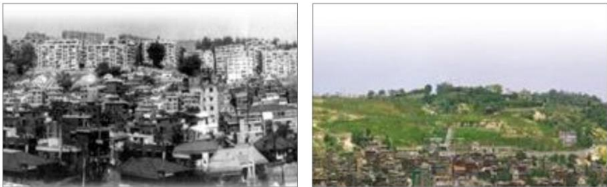
<Figure 9> Naksan Park (Before & After Construction)
