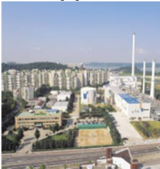
<Mok-dong Cogeneration Plant>
