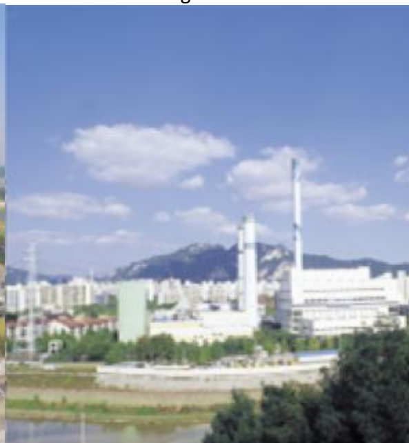
<Nowon Cogeneration Plant>
