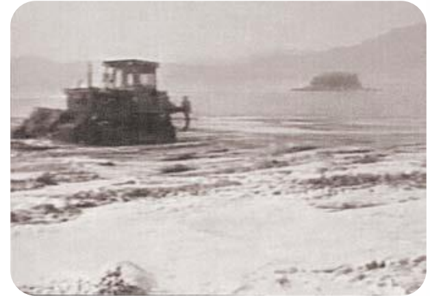
Reclamation work of Landfill ( 1987)
