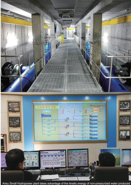
Arisu Small Hydropower plant takes advantage of the kinetic energy of non-pressurized water produce in the Amsa purification center and Noryangjin reservoir. For the first time in Korea, Arisu SHP uses waterwheel installed in the drinking water supply network to produce hydropower.
