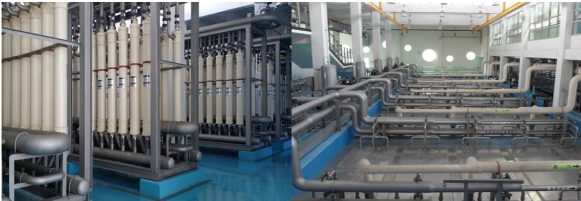
Membrane filtration water purification treatment (pressurized, immersed)
